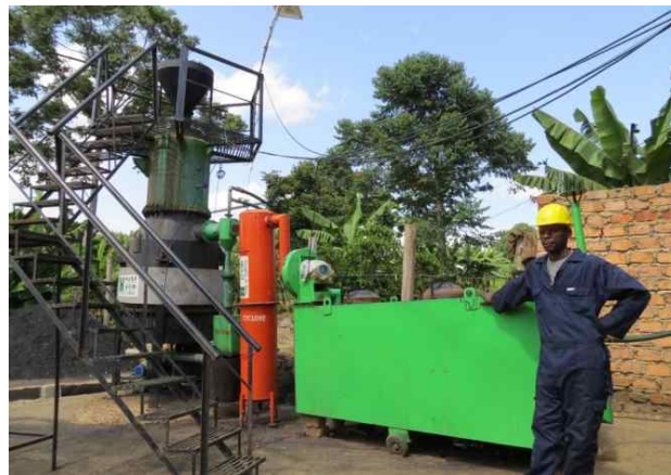
Figure 8 Biomass gasification power plant in a microgrid operated by Pamoja Energy Ltd
