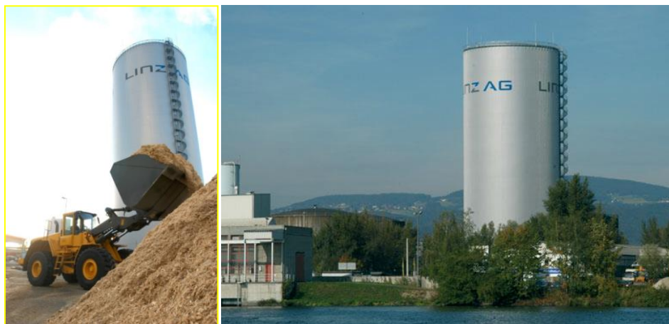
Figure 1: short term thermal storage in the Linz DH network
