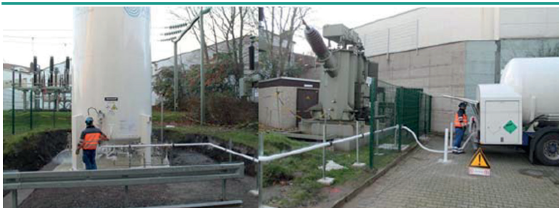
Figure 18: Filling the tank with liquid nitrogen. Photo Courtesy of RWE.
