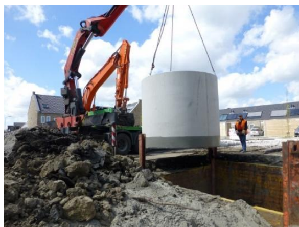
Figure 29. Installation of ice/water storage tank Goes, Province Zeeland, courtesy Marsaki/RWS Partner in Wonen
